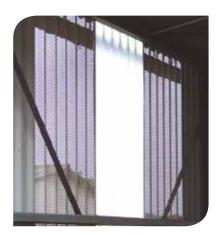
Perforated cladding allows light to enter and provides permanent ventilation in buildings.
